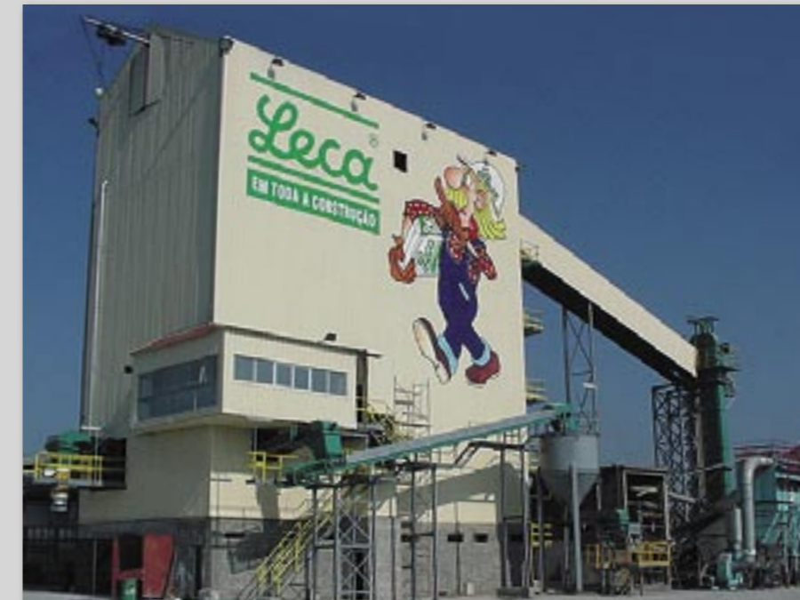
Material fed and discharged to individual to high level bins plus truck loading system.
